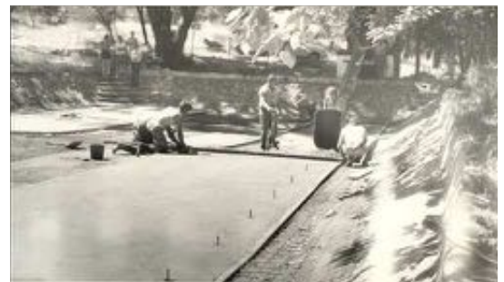
Workmen cementing the pool base in 1972 (Photo: HHS 006852).
